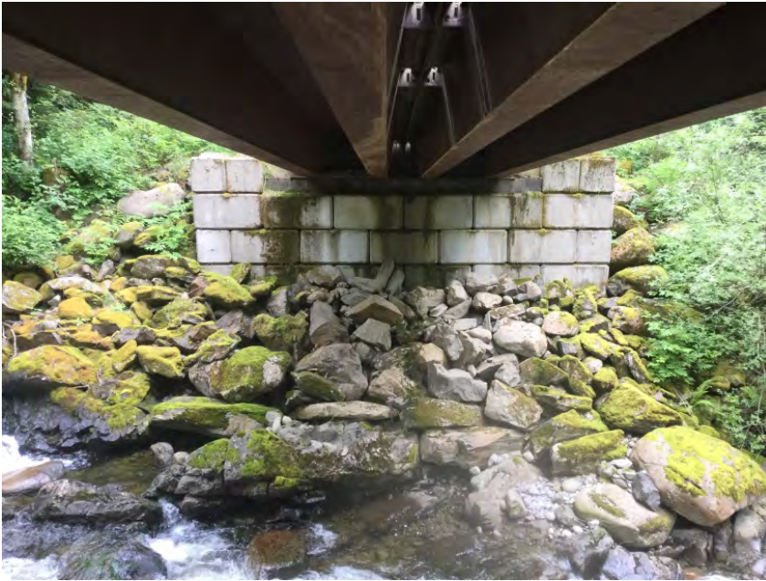
Left Bank Abutment when facing downstream
