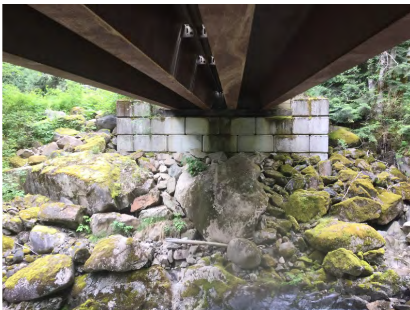
Right Bank Abutment when facing downstream
